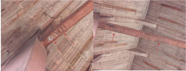
Photo 1-11: Spalling with exposed reinforcement in the transverse beam at the north side of Bent 9.
