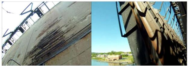
Photo 4-13: Area of heavy spalling with large quantity of exposed rebar on pocket wall at chute 89 on the south side.
