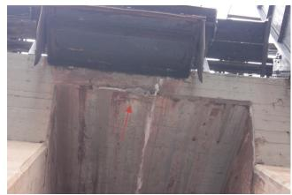
Photo 6-13: Delamination cracking and spalled concrete at overhang between Bents 59 and60 on north side of ore dock.
