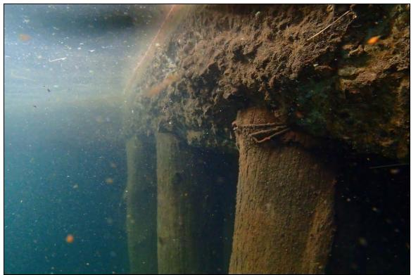
Photograph 11: View of loss of bearing at Piles 9 through 11I in Section 3.
