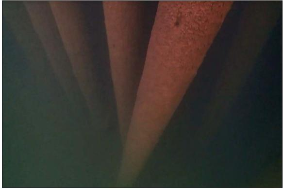
Photograph 20: View of out of plumb Pile 6R in Section 2.
