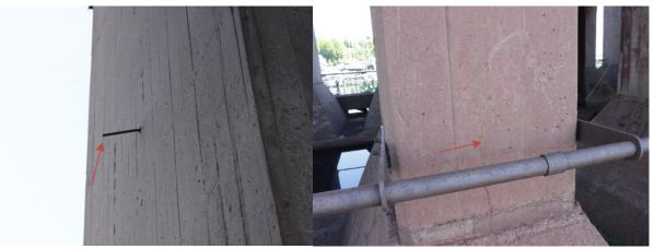
Photo 2-9: Protruding steel bar from the face of Bent 14 on the south side of the dock.
