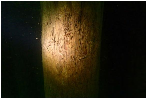
Photograph 9: View of abrasion damage at Pile 33J in Section 7.
