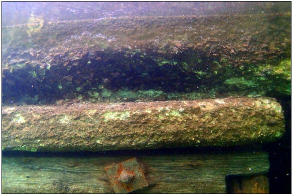
Photograph 25: View of typical concrete spalling above the timber cribs on the north side between Sections 5 and 6.
