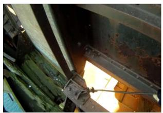
Photo 2-23: View of pocket gate, showing hoist connection on gate and gate guides. Note condition of walkway between chutes.
