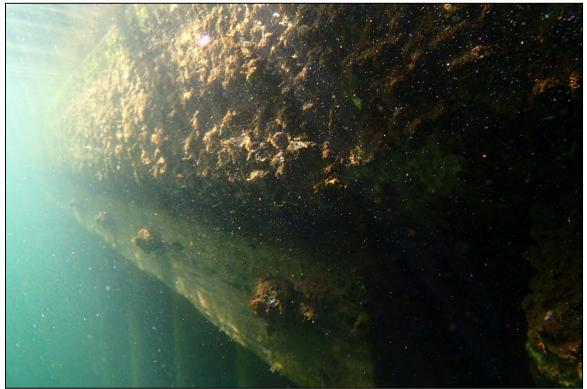
Photograph 24: View of typical concrete scaling on north side of Section 2, looking southeast.
