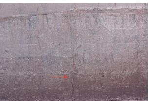
Photo 2-6: Shrinkage cracking on Bent 23 base on south side of dock.
