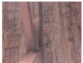
Photo 6-12: Minor honeycombing and exposed rebar in north side of ceiling between Bents 60 and 61.
