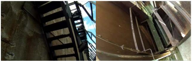
Photo 1-27: View of upper portion of southwest stairs. Note spalled concrete and exposed rebar on pocket wall.
