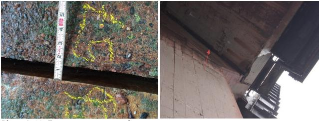
Photo 9-11: Expansion joint on pile cap floor between sections 5 and 6. Note no expansion joint material contained within joint.
