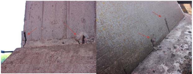
Photo 3-5: Delaminations and spalling on the bottom of Bent 34 located on the north side of the dock.
