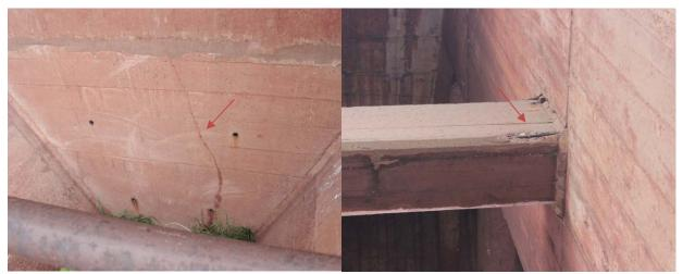
Photo 5-7:Vertical cracking in Bent 52.
