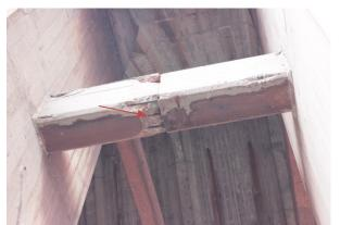
Photo 1-10: Spalling with exposed reinforcement between Bents 5 and 6 on the north side. Note the cold joint mid-span on the beam.
