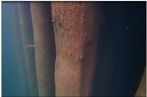
Photograph 19: View of abrasion damage at Pile 40R in Section 3.
