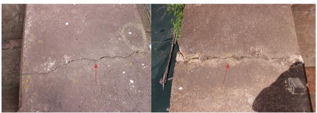
Photo 7-1: Shallow cracking on north side of fender between Bents 72 and 73.
