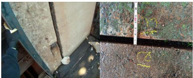
Photo 9-1: View of the expansion joint between Sections 1 and 2 from the walkway on the south side of the structure. Note presence of expansion joint material.
