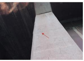
Photo 2-7: Spalls on Bent 23 on the north side of the dock.
