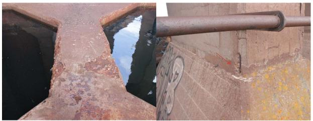
Photo 5-3: Spalling on pile cap floor between Bents 52 and 53.
