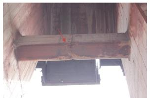
Photo 1-9: Spalling with exposed reinforcement between Bents 5 and 6 on the south side. Note the cold joint mid-span on the beam.
