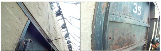
Photo 2-19: Pocket wall where superficial thin spalls and rebar is apparent.
