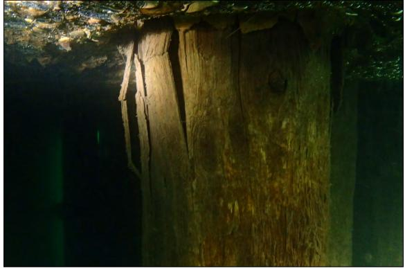
Photograph 10: View of crushed Pile 30J in Section 7.
