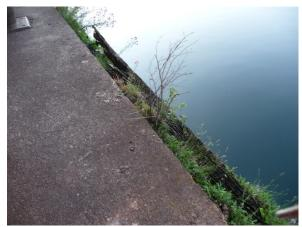
Photo 1-3: Brush and vegetation growing in rotten timbers on fenders.
