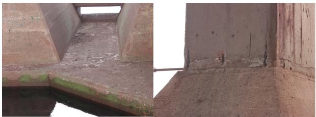
Photo 4-5:Construction joint in pile cap floor between Bents 40 and 41.
