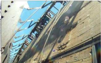
Photo 7-14: View of pocket wall at chute 149 on the south side of the dock showing large area of spalling with exposed rebar.
