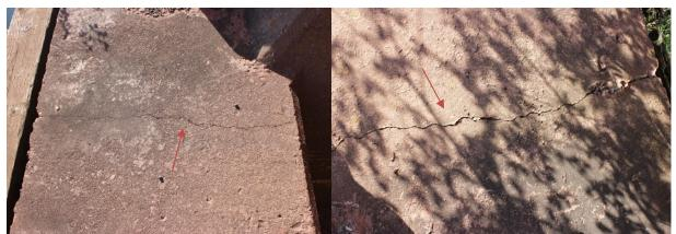
Photo 4-1: Crack in fender between Bents 36 and 37 on the north side of the dock.
