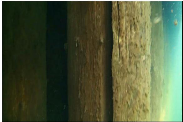
Photograph 22: View of split in Pile 35A in Section 7.
