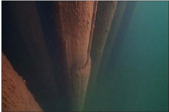
Photograph 18: View of loss of outer shell at Pile 40R in Section 6.
