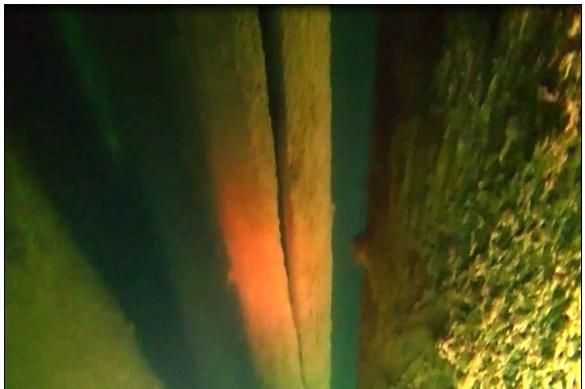
Photograph 17: View of split at Pile 25Q in Section 7.
