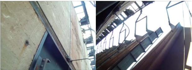
Photo 3-17: Pocket wall where superficial thin spalls and rebar is apparent.
