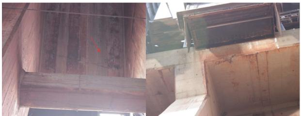
Photo 4-11: Horizontal cracking in ceiling between Bents 39 and 40 on the south side of the dock.
