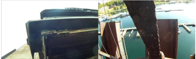
Photo 1-23: Close-up view of the underside of chute 1 showing hinge pin connection.
