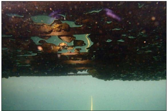
Photograph 28: View of concrete spalling at fifth transverse concrete section in Section 2. Note the air bubbles trapped on the underside of the deck.
