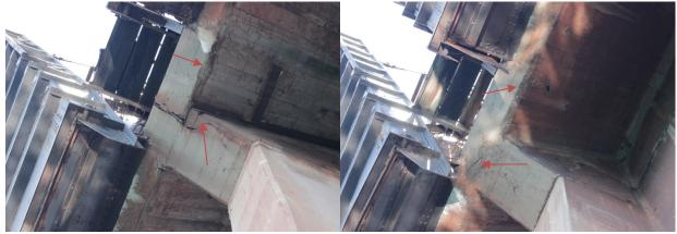
Photo 2-17: Cracking on chute base of Bent 23 near the expansion joint on south side.
