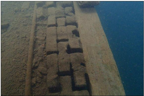
Photograph 7: Typical Wakefield Sheeting configuration of timber crib at interior of Ore Dock.
