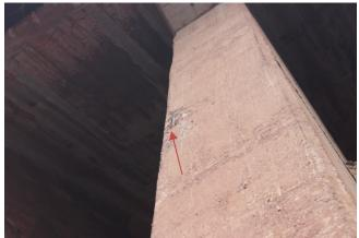
Photo 6-5: Spall with exposed rebar on the south side of ore dock between Bents 59 and 60.
