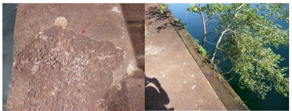
Photo 7-3: Scaling on south side fender between Bents 69 and 70.
