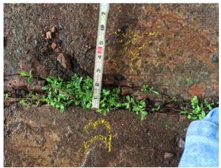
Photo 9-5: Expansion joint on pile cap floor between Sections 2 and 3. Note debris and vegetal growth within joint.
