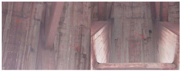
Photo 5-11: Horizontal cracking on north ceiling between Bents 54 and 55.
