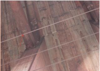
Photo 4-8: Rebar visible on transverse beam between Bents 38 and 39 on the south side of the dock.
