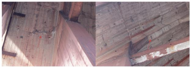
Photo 2-15: Cold joint shown on the expansion joint in this section between Bents 12 and 13 on the north side of the dock.
