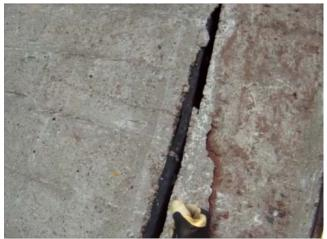
Photo 9-6: View of the expansion joint between Sections 3 and 4 from the walkway on the south side of the structure. Note the joint is open more than the width of the expansion joint material, and presence of delamination in adjacent concrete.
