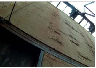
Photo 1-20: Pocket wall showing spalling and rebar.
