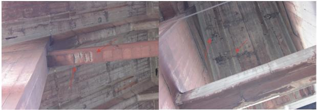
Photo 2-13: Spalls with rebar visible on transverse members, on the north side of Bent 21.
