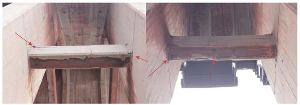
Photo 7-7: Cracking and delaminations in corners of south longitudinal beam between Bents 72 and 73.
