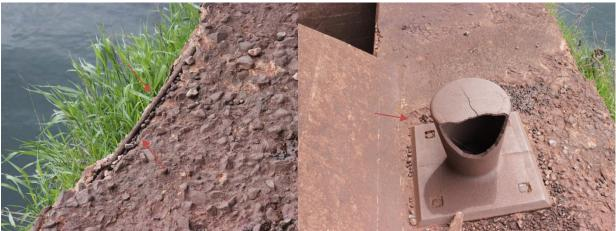
Photo 4-3: Scaling with exposed rebar in fender between Bents 40 and 41 on the south side of the dock. Note missing/rotted timber fender with grass growing in it.
