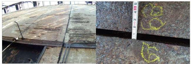
Photo 9-13: Expansion joint on pile cap floor between Sections 6 and 7. Note expansion joint material contained within joint.
