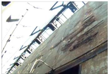
Photo 6-15: View of pocket wall above pocket 111 on the south side of the dock showing large area of spalling with exposed rebar.
