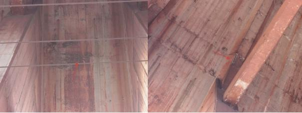
Photo 4-9: Ceiling that contains a cold joint with horizontal cracking and honeycombing between Bents 36 and 37 on the south side of the dock.
