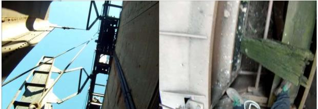
Photo 2-21: Typical view looking up at chutes and hoisting appurtenances.
