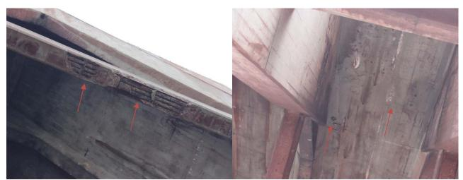
Photo 1-13: Worst-case deterioration observed in the transverse beam at Bent 1.
