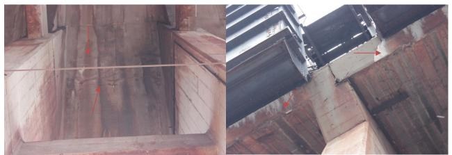
Photo 1-17: Horizontal cracking on ceiling between Bents 3 and 4. Note minor efflorescence.
