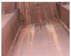
Photo 6-6: View of good condition of shear wall between Bents 62 and 63 on the north side of the ore dock. Note protruding steel bar (possible form tie).
