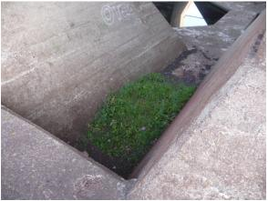
Photo 1-4: Vegetation growing in deposit of iron ore pellets.
