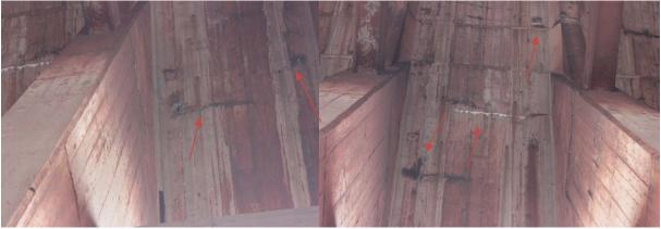
Photo 7-11: Spalls along with horizontal honeycombing along south side ceiling between Bents 69 and 70.
