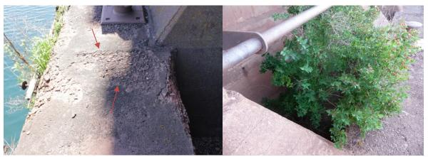
Photo 2-3: Medium-size scaling on north side of fender, between Bents 13 and 14. Note rotten timber fender.
