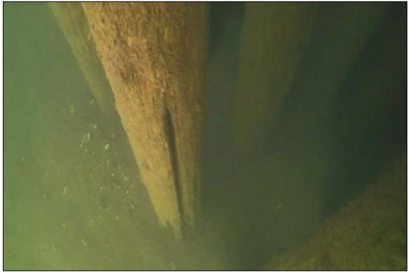
Photograph 16: View of delamination and split at Pile 22R in Section 7.
