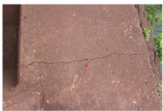
Photo 6-1: Transverse crack in the north fender between Bents 58 and 59.
