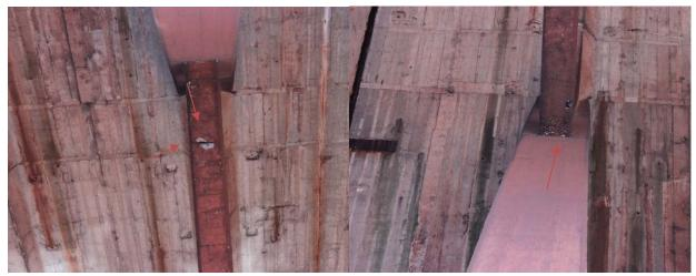
Photo 3-11: Shallow rebar on the underside of the transverse beam on Bent 26.
