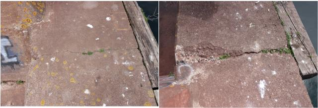
Photo 9-15: Crack in north fender that is serving as the expansion joint between Sections 7 and 8.
