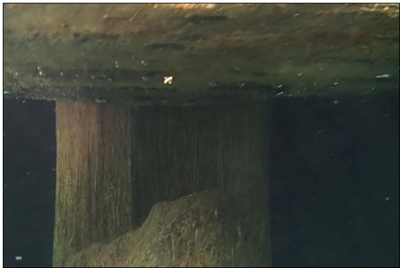
Photograph 21: View of section loss at Pile 39A in Section 4.
