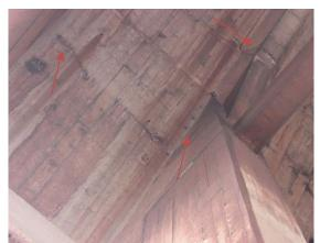
Photo 6-10: Small spalls on south ceiling along with minor honeycombing between Bents 56 and 57.
