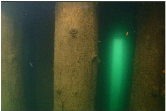
Photograph 5: Typical pile condition below water at interior of Ore Dock, Looking North.
