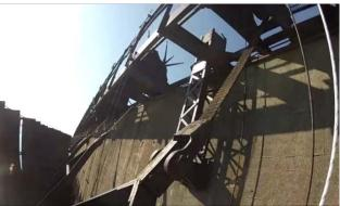
Photo 1-26: Close-up view of hoist belt connection to chute 6. Note good condition of pocket wall.
