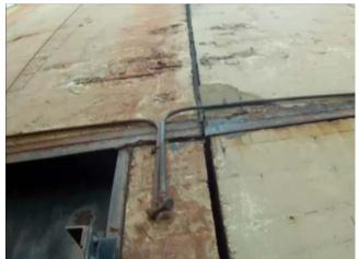
Photo 9-10: View of the expansion joint between Sections 5 and 6 from the walkway on the south side of the structure. Note the joint is open slightly more than the width of the expansion joint material (top), and the joint material has fallen out (bottom).
