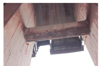
Photo 6-9: Exposed rebar and delamination visible on underside of the north longitudinal beam between Bents 63 and 64.
