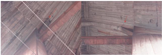
Photo 1-15: Chamfer section of ceiling at south side of Bent 8 showing exposed rebar.
