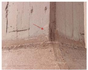
Photo 6-4: Small delamination on south side at the bottom of Bent 57.
