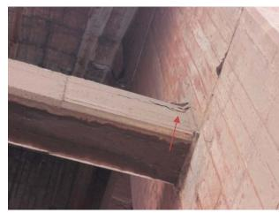
Photo 5-9: Delamination on the south longitudinal beam between Bents 49 and 50.
