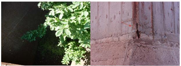
Photo 3-3: Trees growing ina pile of iron ore pellets on pile cap/floor.
