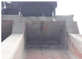
Photo 1-19: View of cracks with efflorescence, with spalling and exposed rebar between Bents 1 and 2, north side.
