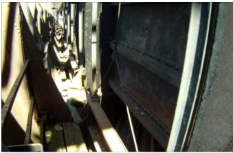
Photo 6-17: View looking down walkway showing the pocket gates, and the bottom of the chutes.
