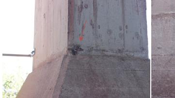
Photo 2-5: Top of bent bases often have small spalls with rebar visible, this one is located on the north side of Bent 17.
