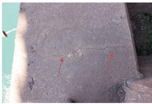
Photo 2-1: This photo shows cracking on the south side of the fender between Bents 14 and 15.
