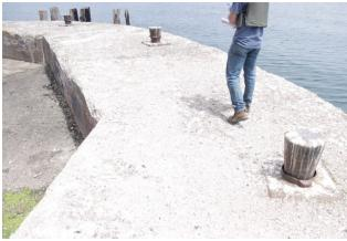
Photo 8-1: Section at the end of the ore dock in which major scaling has taken place.
