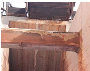
Photo 4-7: Spall with rebar visible on longitudinal beam between Bent 37 and 38 on the north side of the ore dock.
