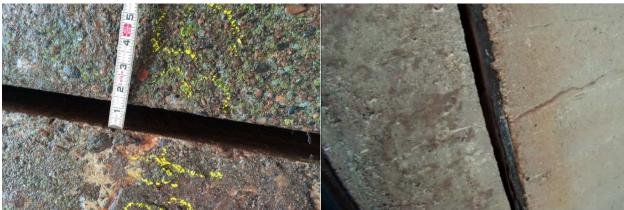
Photo 9-7: Expansion joint on pile cap floor between Sections 3 and 4. Note no expansion joint material contained within joint.
