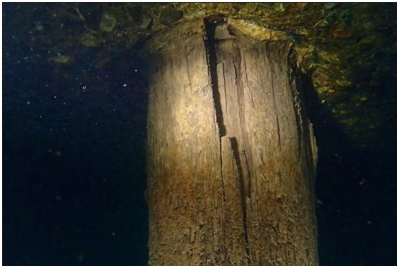
Photograph 13: View of delamination of outer shell at Pile 35I in Section 3.
