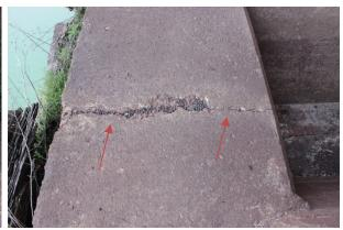
Photo 2-2: Cracking on south side of fender with some spalling coming from the crack, between Bents 17 and 18.
