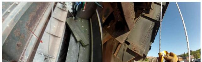
Photo 1-21: Additional steel top member found on pocket doors 1 through 27.
