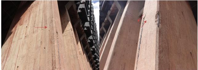
Photo 1-7: Delamination/spalling on Bent 9, south side. Note exposed reinforcement with no concrete cover.
