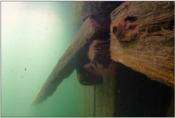
Photograph 23: View of broken timber wale on northeast side of Section 7, looking east.
