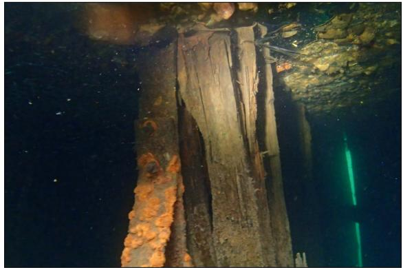
Photograph 12: View of delamination of outer shell at Pile 33I in Section 3.
