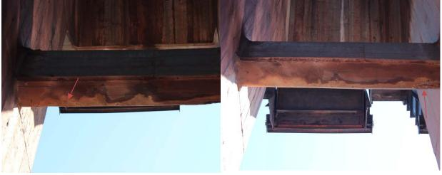
Photo 3-9: Delamination on cross beam between Bents 25 and 26 on the south side of the dock.
