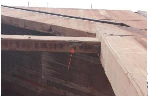
Photo 7-9: Rebar apparent on underside of transverse beam on Bent 76 on the north side of the dock.
