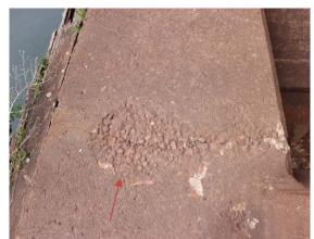
Photo 6-2: Transverse crack and scaling on the north fender between Bents 59 and 60.
