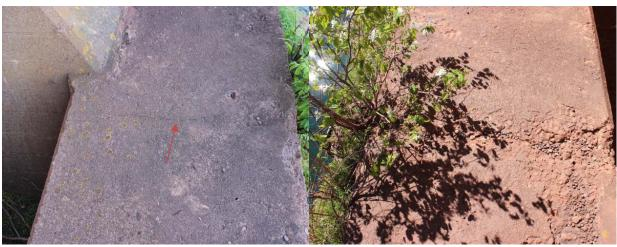
Photo 3-1: Cracking on fender between Bents 25 and 26 on the north side of the dock.
