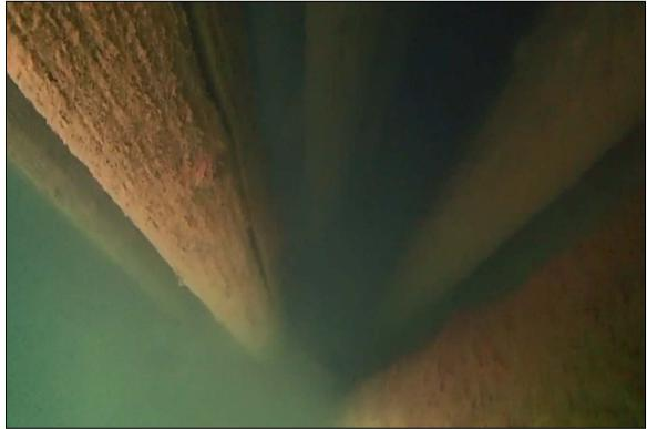
Photograph 14: View of split at Pile 5R in Section 7.
