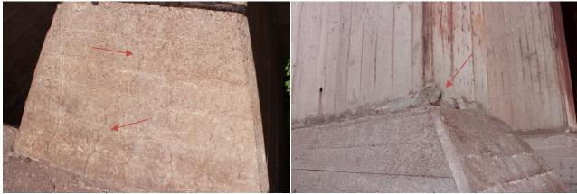
Photo 1-5: Shrinkage cracks on face of south base of Bent 7.
