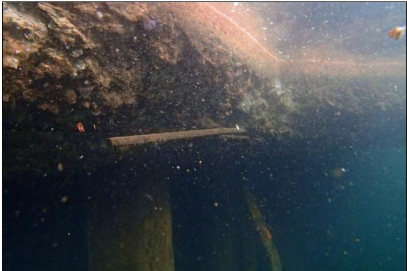
Photograph 27: View of concrete spalling on the north side of Bay 2 in Section 3.
