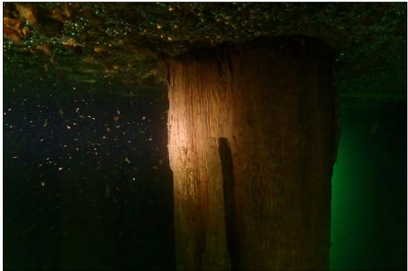
Photograph 8: View of delamination of outer shell at Pile 35J in Section 7.
