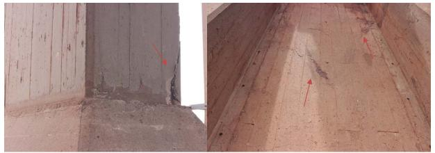
Photo 7-5: Spall on south base of Bent 68 exposing rebar.
