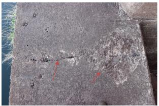
Photo 1-2: Shrinkage crack in walkway between Bents 2 and 3, on the south side of the dock. Note localized surface scaling.
