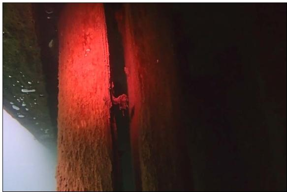
Photograph 15: View of split at Pile 19R in Section 7.
