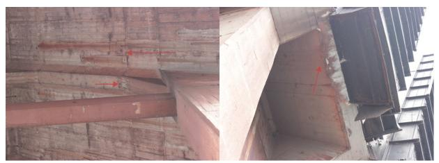
Photo 5-13: Rebar visible in the chamfer section of the south side of the ceiling on Bent 47.
