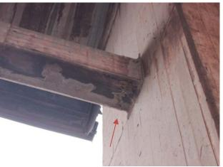
Photo 5-10: Delamination cracking on the north longitudinal beam between bent 49 and Bent 50.
