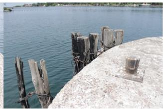
Photo 8-2: Piles at the end of the ore dock that have become rotten and loose.
