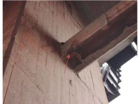
Photo 6-8: Spall with exposed rebar and cracking in corner of longitudinal beam between Bents 59 and 60 on the north side of dock.
