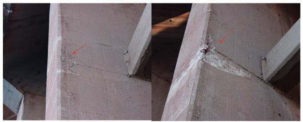
Photo 3-7: Delaminations on Bent 29 on the north side of the dock.
