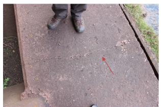
Photo 1-1: Shrinkage crack in walkway between Bents 10 and 11, on the north side of the dock. Note deteriorated timber bumper.
