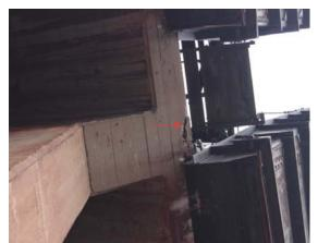
Photo 6-14: Small delamination of concrete on the chute base between Bents 59 and 60 on the south side of the dock.
