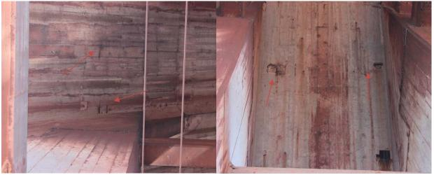
Photo 3-13: Rebar visible on ceiling between Bents 24 and 25 on south side of dock.
