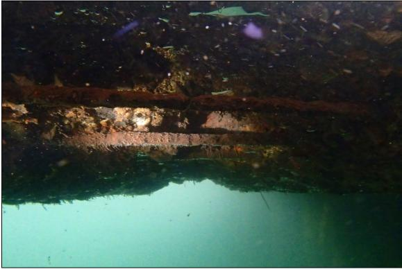
Photograph 26: View of concrete spalling at second transverse concrete section in Section 5.
