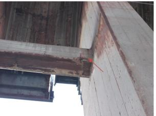
Photo 2-11: Delamination cracking in the longitudinal beam between Bents 15 and 16 located on the north side of the dock.
