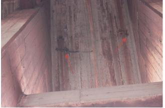
Photo 6-11: Minor honeycombing and exposed rebar on north side ceiling between Bents 63 and 64.
