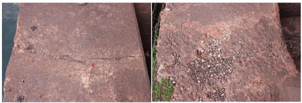
Photo 5-1: Crack in fender between Bents 49 and 50 on the south side of the dock.
