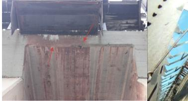
Photo 7-13: Chute base with minor cracking with exposed rebar between Bent 70 and 71 on south side of dock.
