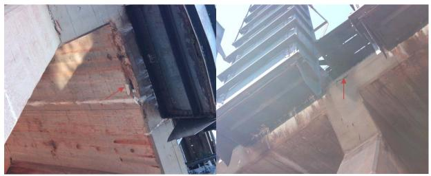
Photo 3-15: Spalls with shallow rebar on overhang between Bents 27 and 28 on the north side of the dock.
